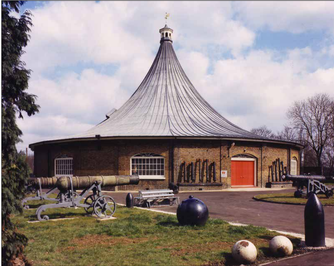
Fig. 53 The Rotunda from the south-west on 9 April 1975, following the completion of the extensive restoration programme. (© Crown copyright. Historic England Archive, ref. p_g21156_003)
