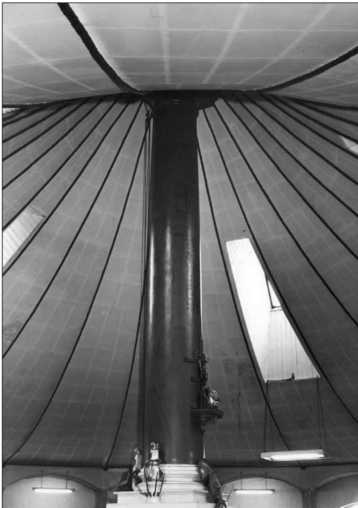
Fig. 55 The Rotunda's canvas ceiling on 6 April 1971, before 'restoration'. This fabric roof lining, with its radiating ropes, was probably to a large extent that erected by John Nash and his workmen at Carlton House in 1814 and re-erected at Woolwich in 1819-20. Compare George Scharf's painting of 1828 (see Fig. 20). (© Crown copyright. Historic England Archive, ref. p_g15031_007)
