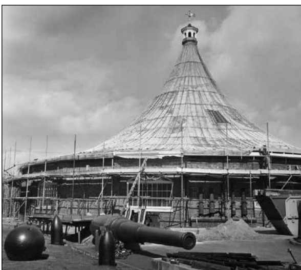
Fig. 52 The Rotunda at the start of repairs to the roof, on 5 April 1973, and before the removal of the Victorian rooflights. (© Crown copyright. Historic England Archive, ref. p_g19054_007)
