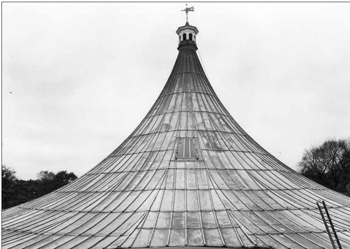
Fig. 36 The lead roof of the Rotunda, almost certainly dating from works undertaken in 1862-3. Four roof lights were inserted at this time. The roof was reclad and the windows removed in 1973-74, soon after this photograph was taken on 17 October 1972. Traces of the wartime camouflage paint are still visible. (© Crown copyright. Historic England Archive, ref. p_g18526_013)
