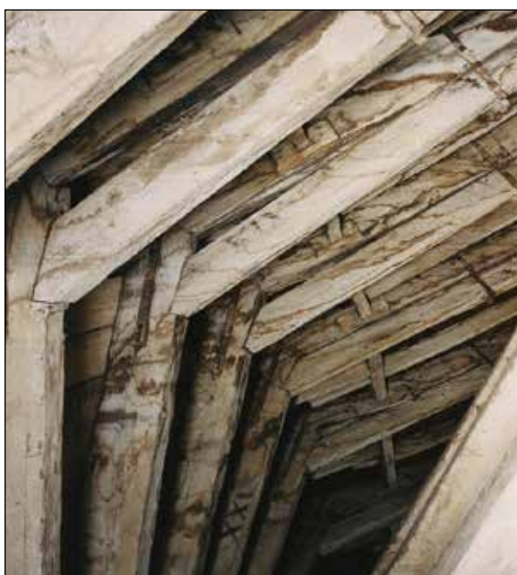
Fig. 50 The original roof structure of the Rotunda surviving above the replaced canvas lining, 24 July 2004. (© Historic England Archive, aa048107)
