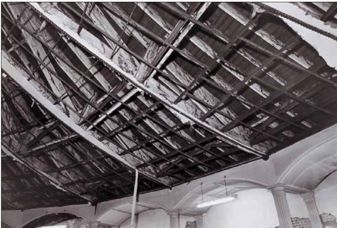
Fig. 27 The internal framework of the roof of the Rotunda during restoration, 17 October 1972, with the nineteenth-century boarded outer covering visible above. (© Crown copyright. Historic England Archive, ref. p_g18526_007)
