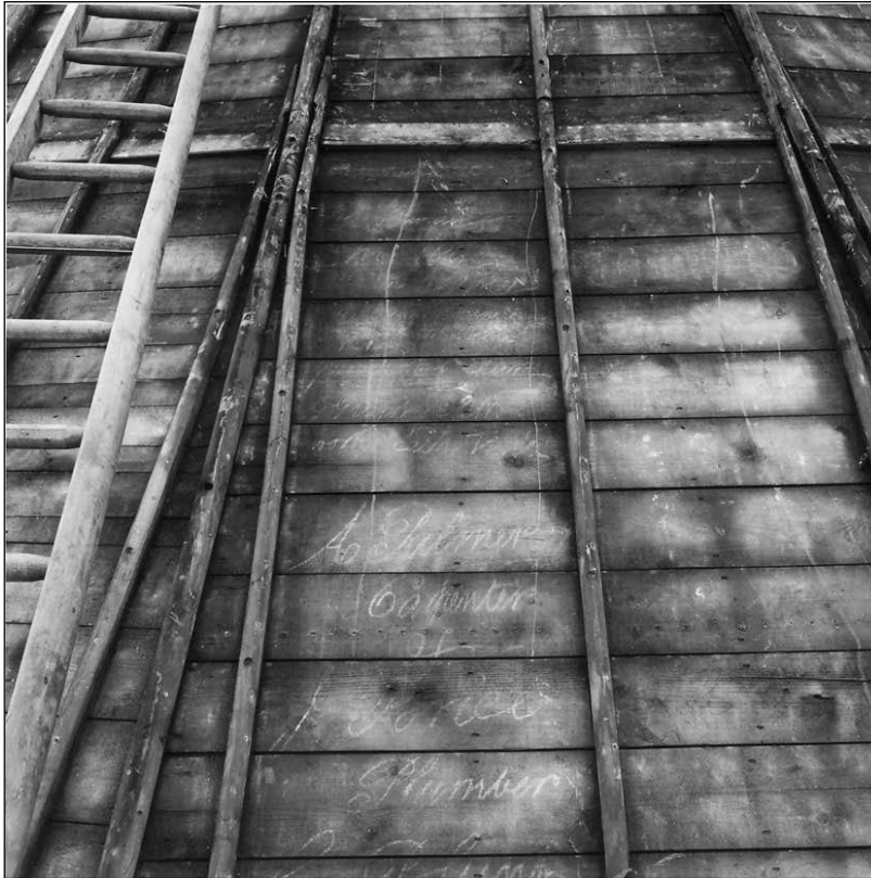
Fig. 26 Detail of the boarding exposed beneath the lead cladding, 9 October 1973. The boards are marked in chalk with the names of the workmen, including a carpenter and a plumber, probably employed during the Rotunda's re-erection in 1819-20. (© Crown copyright. Historic England Archive, ref. p_g19692_006)
