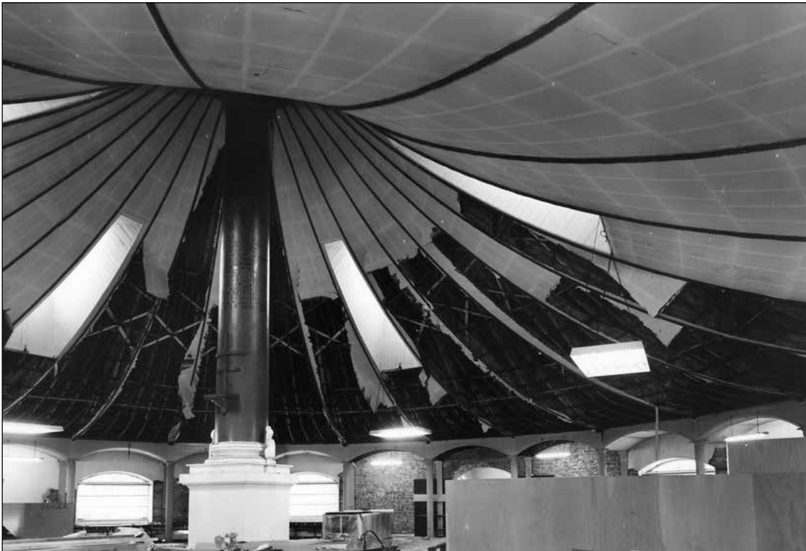
Fig. 48 The removal of the fabric lining of the Rotunda's roof, 17 October 1972. This canvas may have dated to the time of the building's original construction in the gardens of Carlton House in 1814, if not to the time of its re-erection at Woolwich in 1819-20. (© Crown copyright. Historic England Archive, ref. p_g18526_018)
