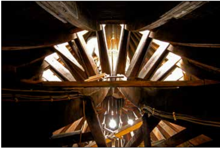
Fig. 70 View towards the apex of the laminated timber roof over the Music Room at the Brighton Pavilion. The inclined members are the array of upper struts, joining the upper and lower chords. (© Historic England, Derek Kendall)
