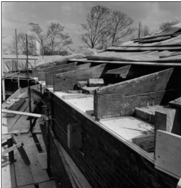
Fig. 51 Repairs to the leadwork of the Rotunda’s roof being undertaken, 5 April 1973. (© Crown copyright. Historic England Archive, ref. p_g19054_004)
