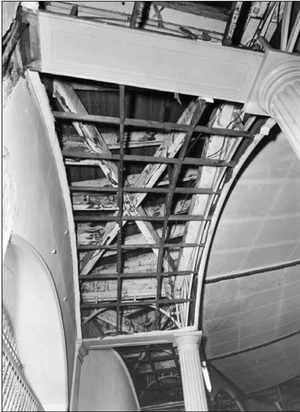
Fig. 47 The exposed roof structure following the removal of the canvas covering above the Rotunda's alcoves, 17 October 1972. (© Crown copyright. Historic England Archive, ref. p_g18526_017)
