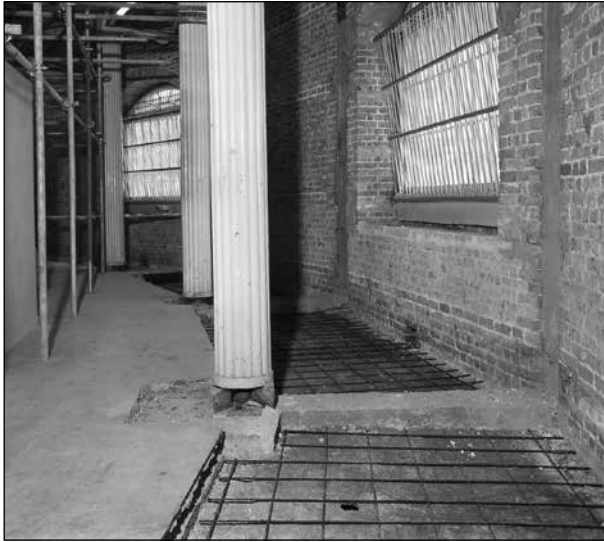
Fig. 44 Installation of the concrete floor at the Rotunda, 5 April 1973. (© Crown copyright. Historic England Archive, ref. p_g19054_008)
