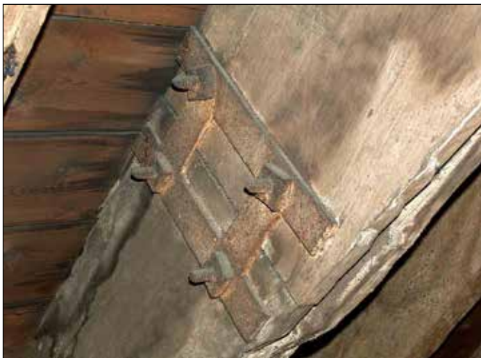
Fig. 64 Forged-iron fishplate in the roof of the Rotunda, used here to splice the laminated timber upper chord. (© Historic England, Jonathan Clarke)
