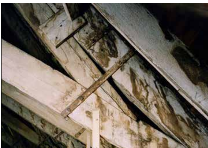
Fig. 65 Inverted U-shaped iron stirrup in the roof of the Rotunda, fastening the laminated upper chord to two struts. (© Historic England Archive, Patricia Payne, ref. aa048109)
