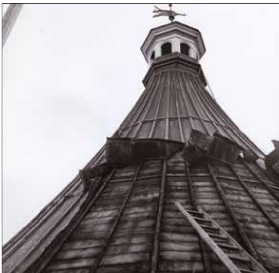
Fig. 25 Photograph of October 1973 showing the exposed timber underlay of the roof of the Rotunda during ‘restoration’. The boarding probably dates from the building’s re-erection in Woolwich, 1819-20. (© Crown copyright. Historic England Archive, ref. p_g19692_010)
