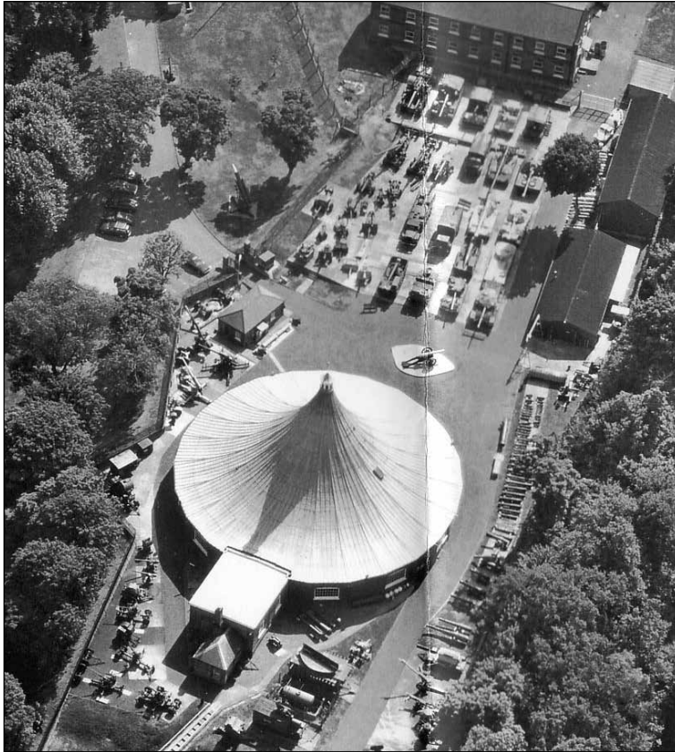
Fig. 37 Aerial photograph of the Rotunda, 2 September 1994. Work dating from the early 1860s includes the lead roof (repaired in the 1970s, when the windows were removed) and the north extension, visible at the bottom of the picture. (© Crown copyright. Historic England Archive, ref. nmr_15157_52)
