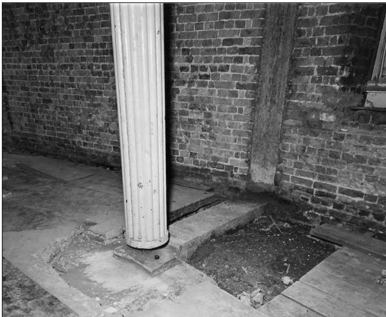
Fig. 43 Photograph of 17 October 1972 showing one of the Rotunda’s timber wall posts and part of its wooden floor before removal as part of restoration. (© Crown copyright. Historic England Archive, ref. p_g18526_001)
