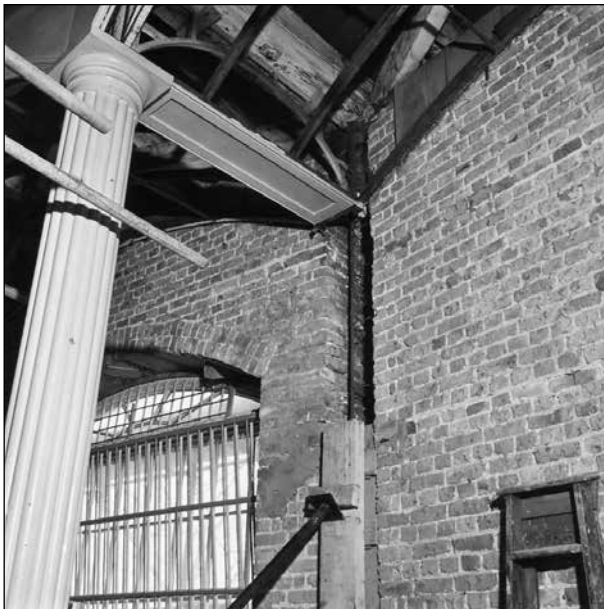
Fig. 45 The exposed wall and roof structure at the perimeter of the Rotunda after the removal of an embedded timber wall post, and during installation of a new reinforced concrete post, 7 March 1973. (© Crown copyright. Historic England Archive, ref. p_g18760_002)
