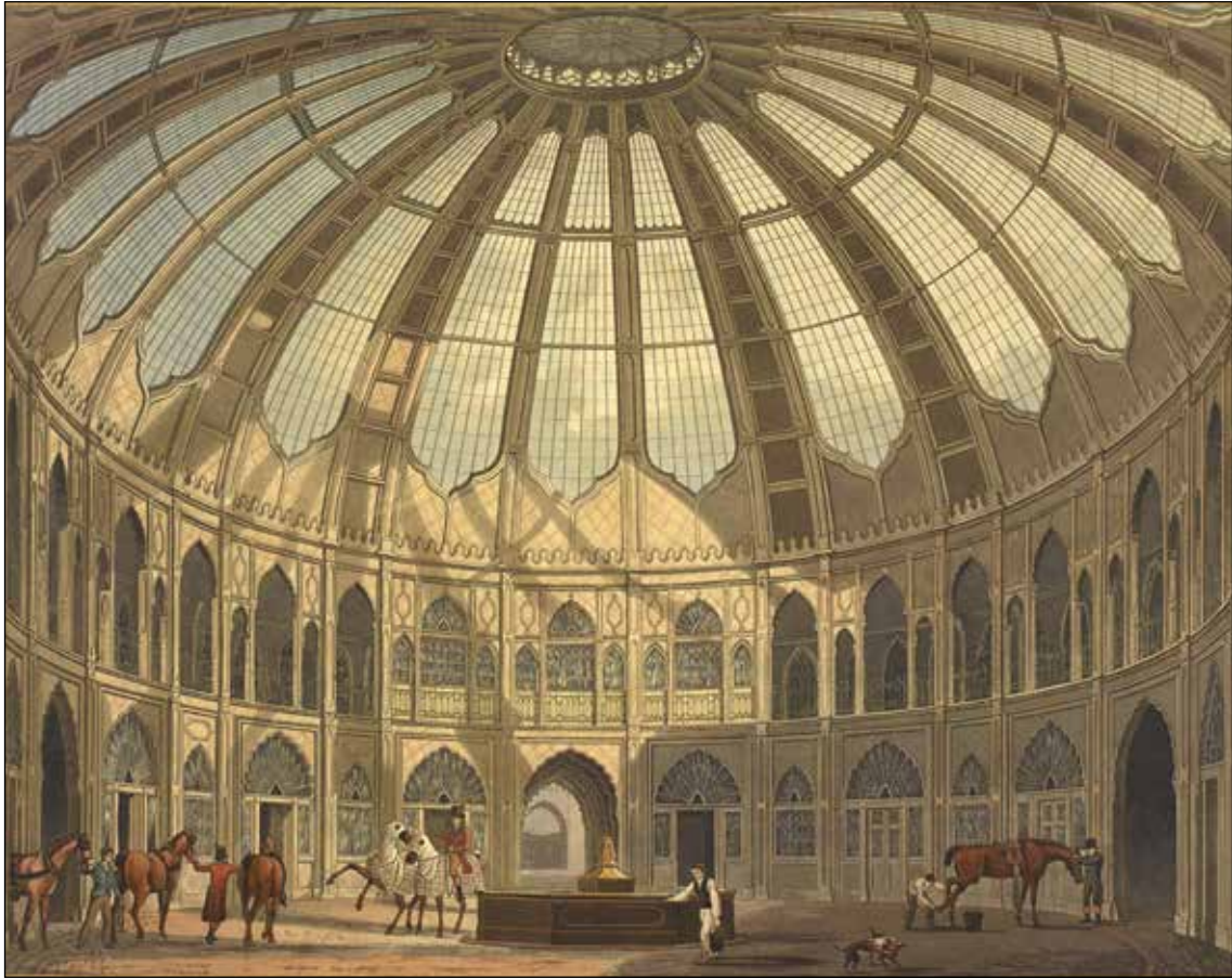
Fig. 71 The central rotunda of William Porden's Riding School and Stables, built 1804-8, as illustrated in John Nash's The Royal Pavilion at Brighton (1827). This dome was probably the first large-scale use of laminated timber in Britain. The building was converted for public use, incorporating a museum, gallery and concert hall, in 1867-73 and is now named 'the Dome'. (© The British Library Board, 557*.h.19, p. 26)
