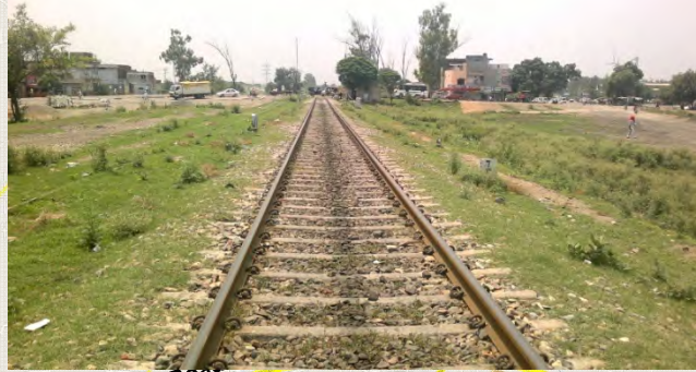
Verka Railway Crossing
