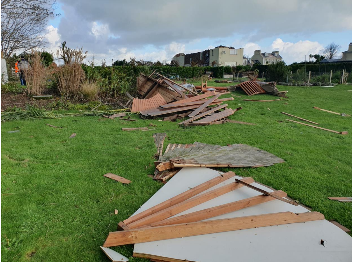
Figure 48: Debris from Greencliff cottages, Fliquet. View looking to the north-west.
