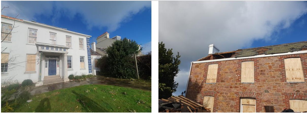
Figure 49: Damage to neighbouring properties in Fliquet.
