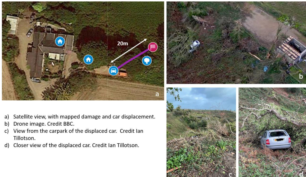
Figure 43: Overview map and photographs of a displaced car at St. Catherine's Woods.
