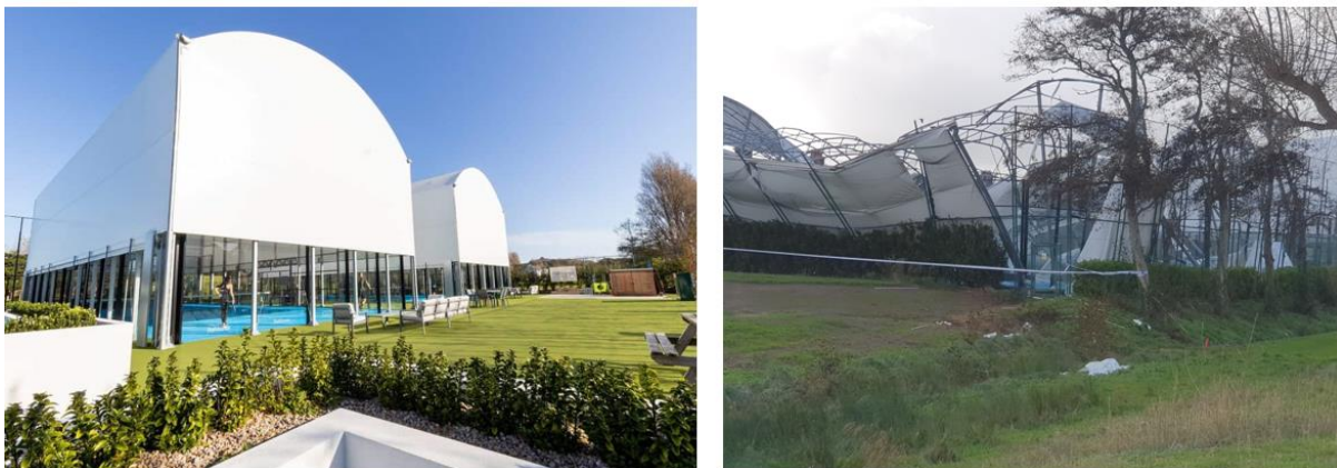
Figure 18: Island Padel sports pavilion was badly damaged. (Before image included for comparison).
