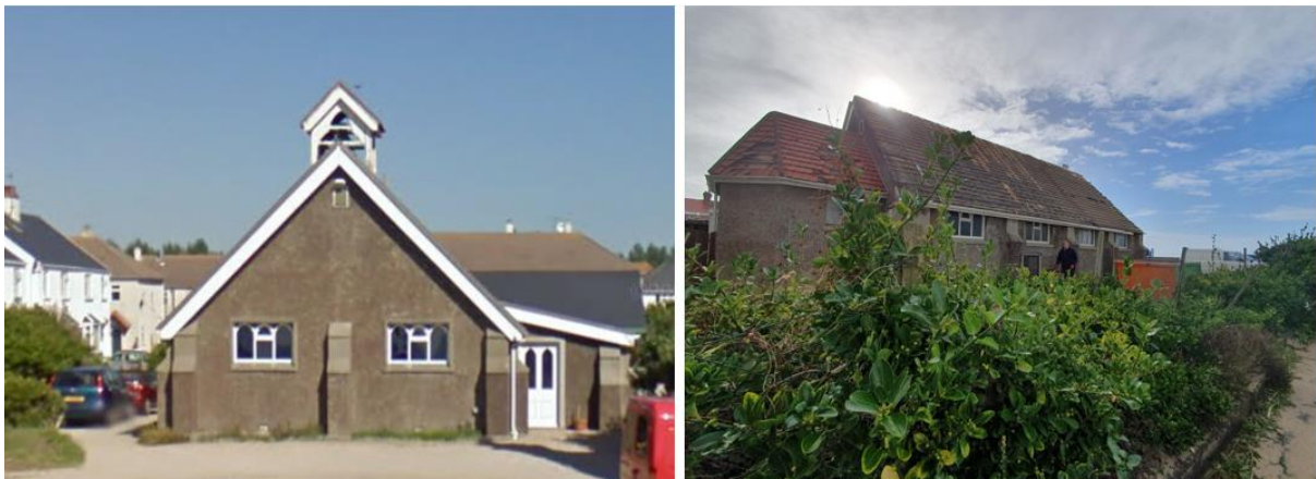
Figure 7: St Nicholas Church, St Clement. Before (looking from the south) and after (looking from the west).
