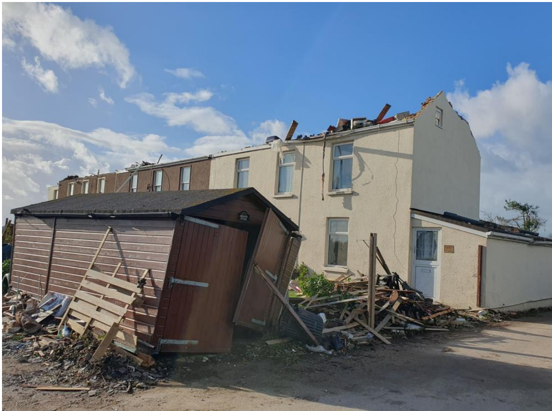
Figure 46: View of western face of Greycliff Cottages, Fliquet.
