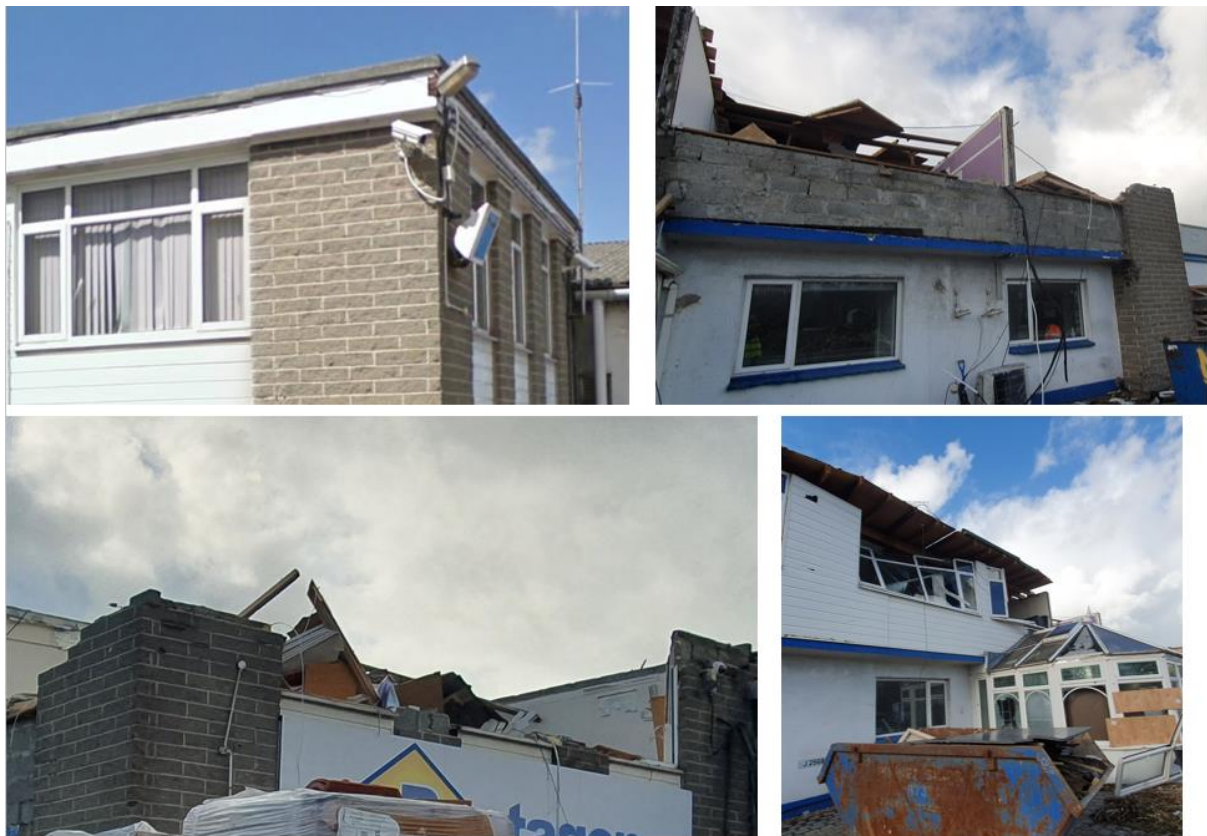
Figure 21: Pentagon Wholesale building, before (top left) and after (remaining photos).
