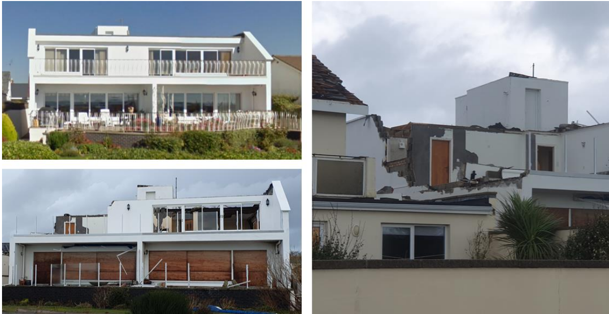
Figure 6: Beach front property in St Clement, before and after. This lost a substantial part of the upper floor as well as the roof. All beachside windows were smashed.
