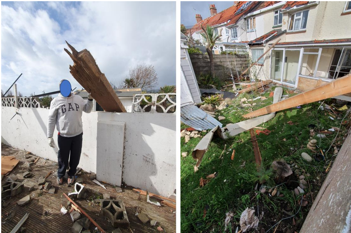
Figure 15: Large beam of wood from the Geoff Reed Table Tennis Centre thrown 150m north-west.
