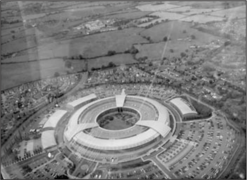
Aerial view of GCHQ - Ron Prewer
