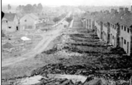
Orchard Avenue under construction 1950/51 (C) M. Holtam
