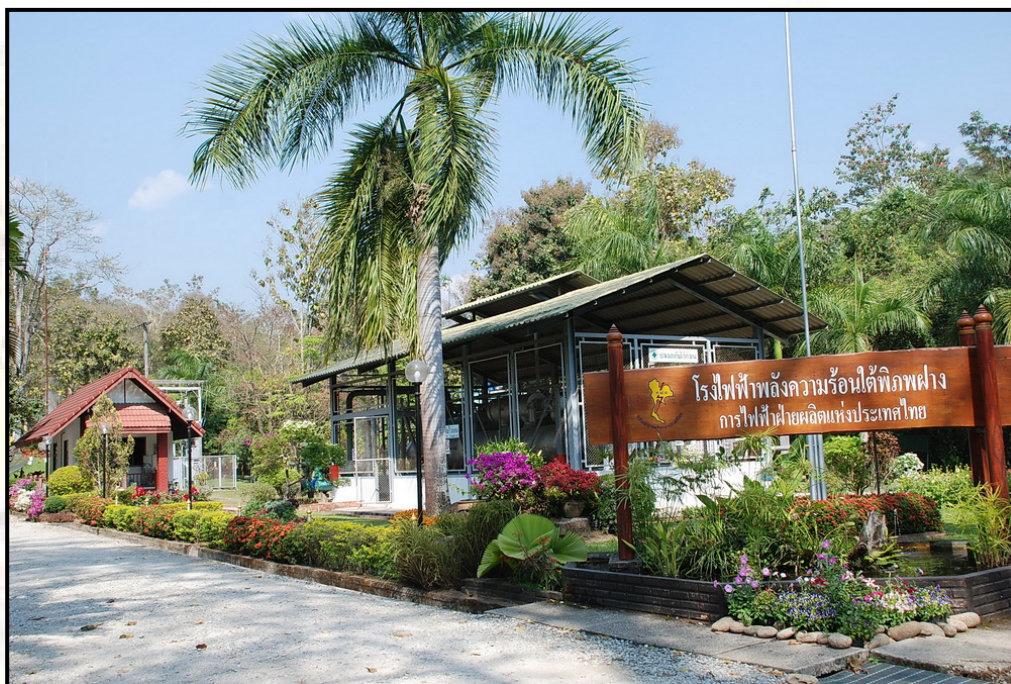
The figure shows 300kW binary cycle geothermal power plant.
