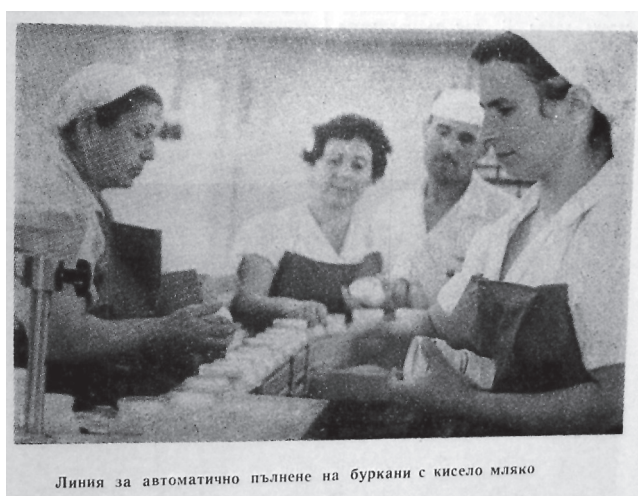
Figure 13 – Productive line for automatic filling of yoghurt jars. Source: Хранителна промишленост 9 (1971): 1 ( Food Industry 9 (1971): 1).
