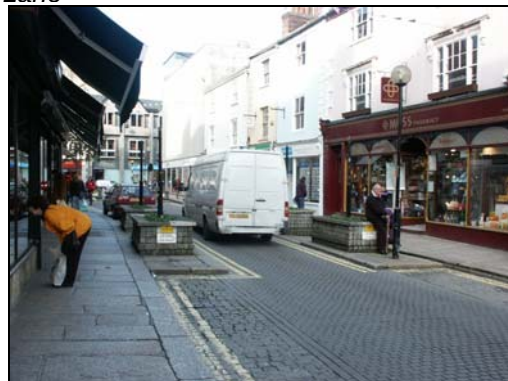
High quality elements of the public realm, such as granite pavements and kennels, are mixed with lower quality materials and clutter. Lower Lemon Street
