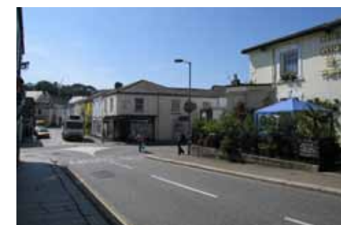
An inconsistent palette with granite paving slabs and kerbs on the left pavement, tarmac carriageway then granite kerbs but with herringbone block paving on the right pavement.
