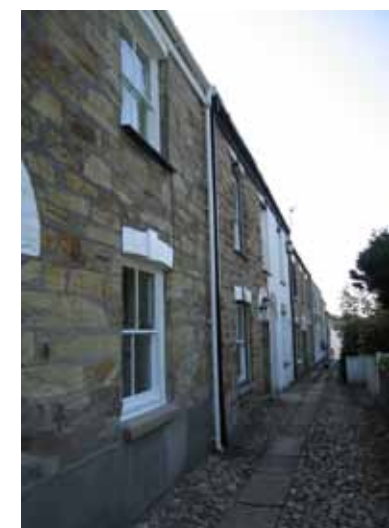
Carclew Terrace fronts a footpath along the contours of the hillside
