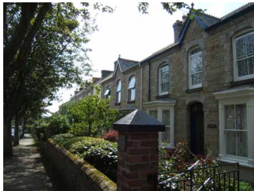
Terraced villas on Carvoza Road
