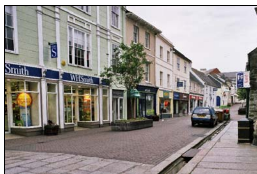
Less individually prominent buildings still display high quality detailing and architectural enrichment, Pydar Street
