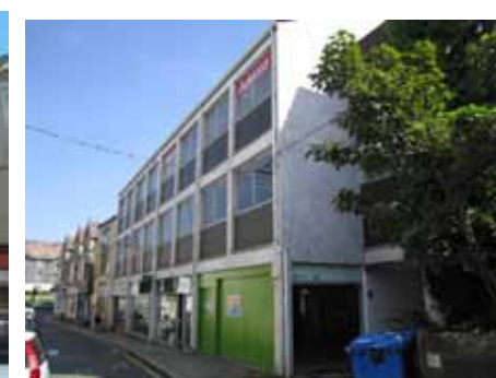
1-4 New Bridge Street
