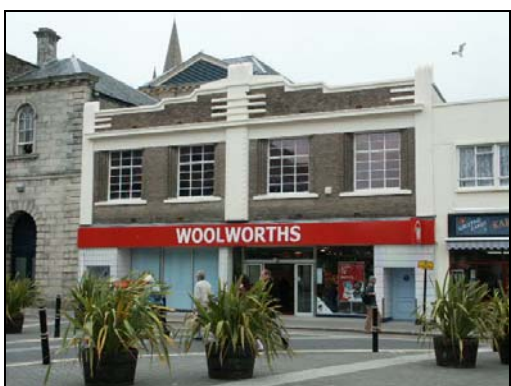
Back Quay elevation of 13-15 Prince's Street. Part of a good group of mid 20 th century buildings.
