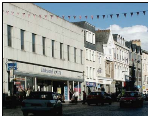
The Littlewoods building, Boscawen Street, an unsympathetic 20 th century addition to the Conservation Area
