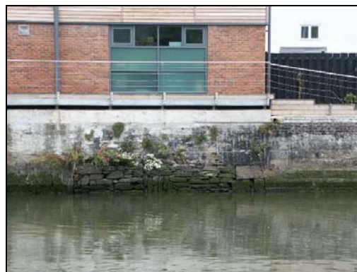
The quay structures themselves contain archaeological sequences of material of interest which could benefit from further investigation
