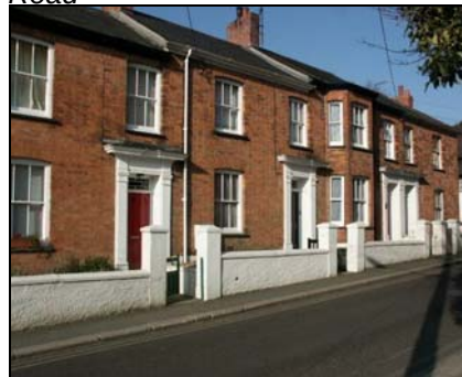
St Mary's Terrace, Kenwyn Road. An unusual red brick terrace with classical detailing
