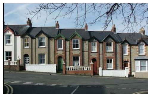
Areas with good historic integrity are important to Truro's character and interest even when individual buildings are not listed. For example Daniell Road
