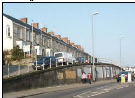
Coronation Avenue is set on a distinctive raised terrace with robust iron railings. Niches for advertising panels were conceived as part of the design of the retaining wall. Standard highway street lighting fails to recognise the surrounding special character
