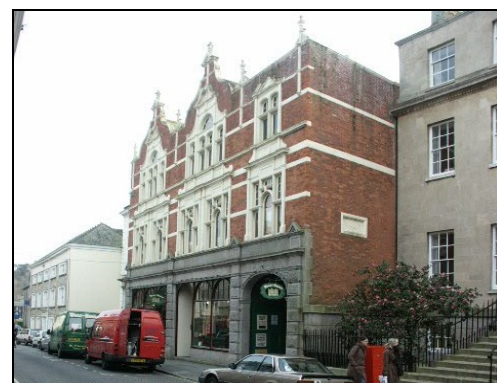
Imported brick and terracotta, Wear House, Prince's Street
