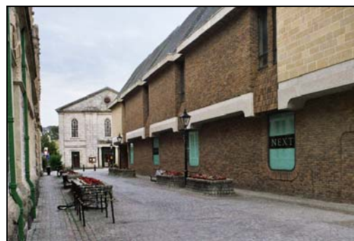
Some twentieth century buildings are unsympathetic to the character of their surroundings. Former Marks and Spencer building Union Place
