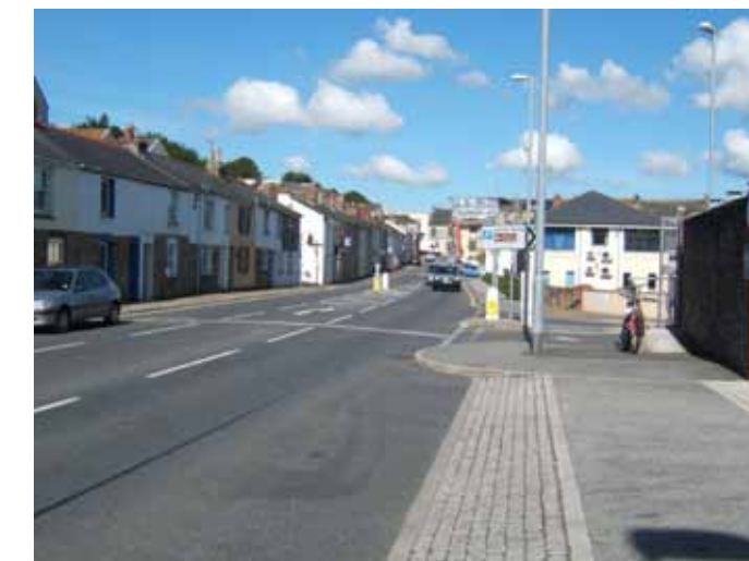
The widening of Fairmantle Street has swept away one side of the terrace.
