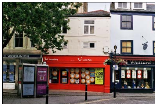
Unsympathetic shop front treatment and partially blocked and grilled first floor windows erode the architectural integrity of this historic building, 2 King Street
