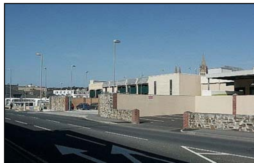
The setting of the Conservation Area includes some of the most damaged areas of townscape, for example Fairmantle Street
