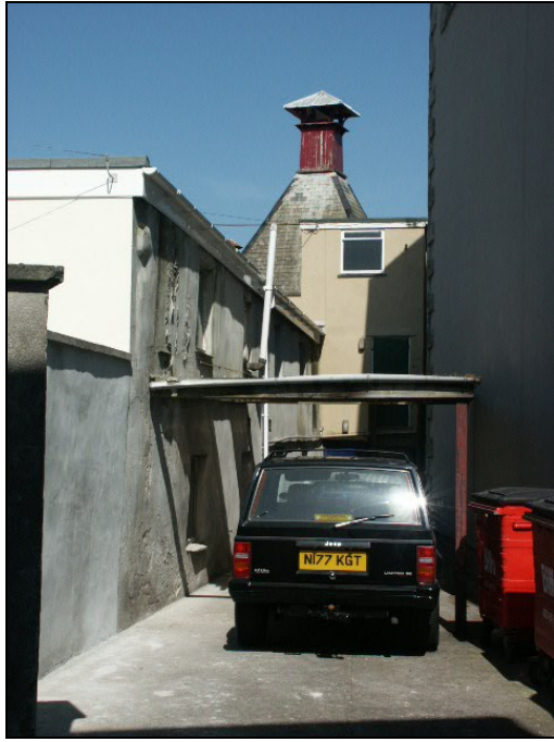
Surviving malthouse located in rear plot of 10 Pydar Street
