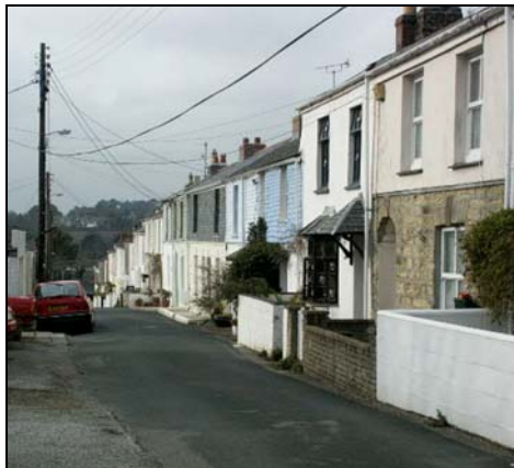
Paul's Row, killas rubble ground floors with slate-hanging or stucco first floors
