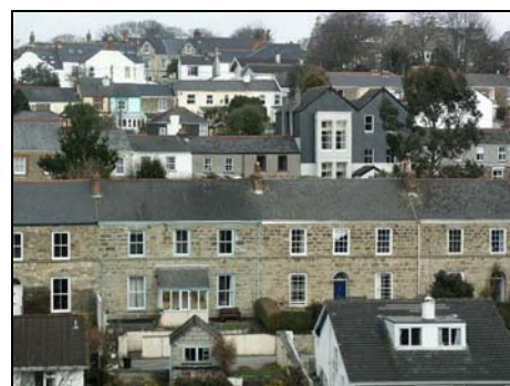
Double fronted properties of Truro Vean Terrace in foreground
