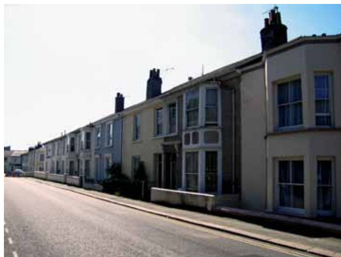
The condition of these properties on St Georges Road diminishes the contribution that they make to the character and appearance of the conservation area
