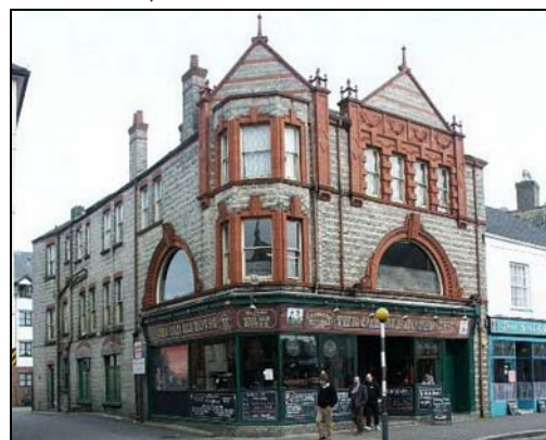
Late Victorian commercial buildings; The Old Ale House originally built as retail premises
