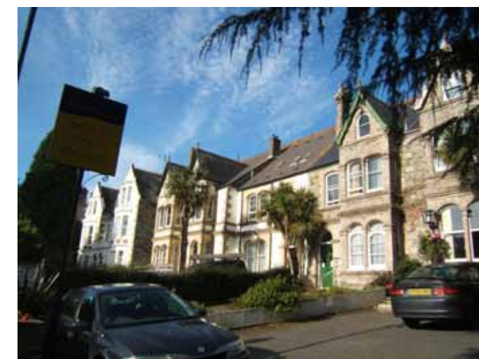
Villa properties on Crescent Road and Falmouth Road set deep within their plots
