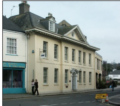
Wealth generated by tin was used to create impressive town houses such as the 'Old Mansion House', Quay Street, of 1709 built for Samuel Enys
