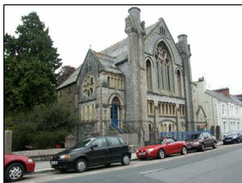
Impressive former Methodist Chapel, St George's Road
