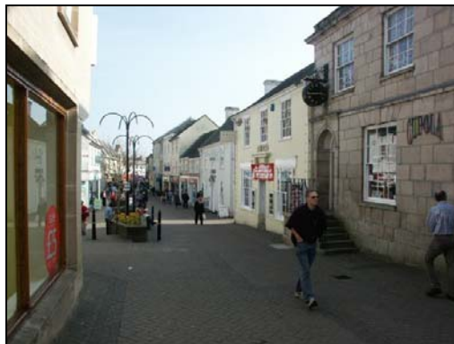
Pydar Street poor public realm treatment
