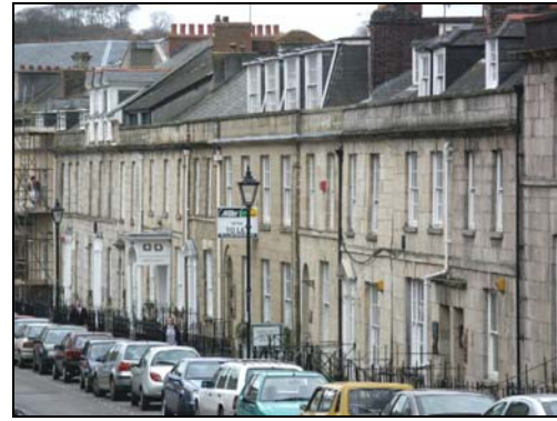
Ashlar façades of Lemon Street
