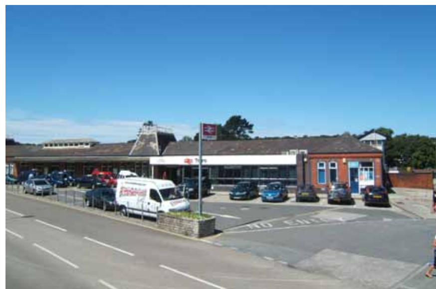
The railway station environment could be improved to provide an attractive welcome to the city.
