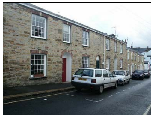
Local killas stone used faced and squared and as irregular rubble. Mortar mixes and application technique are as important in the final appearance as the stone itself. Carclew Street.
