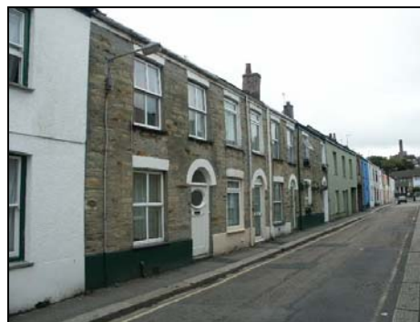
Typical details of round headed doorways and shallow window arches with key stone details, St Dominic Street
