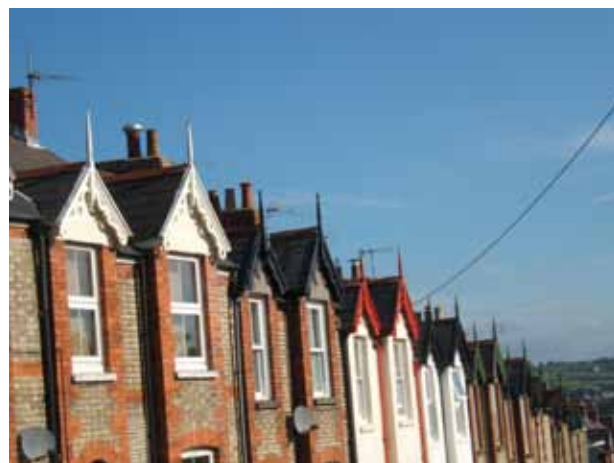
The distinctive roofscape of Daniell Road.
