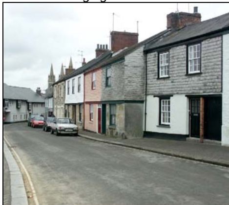
Surviving slate-hung houses, Kenwyn Street
