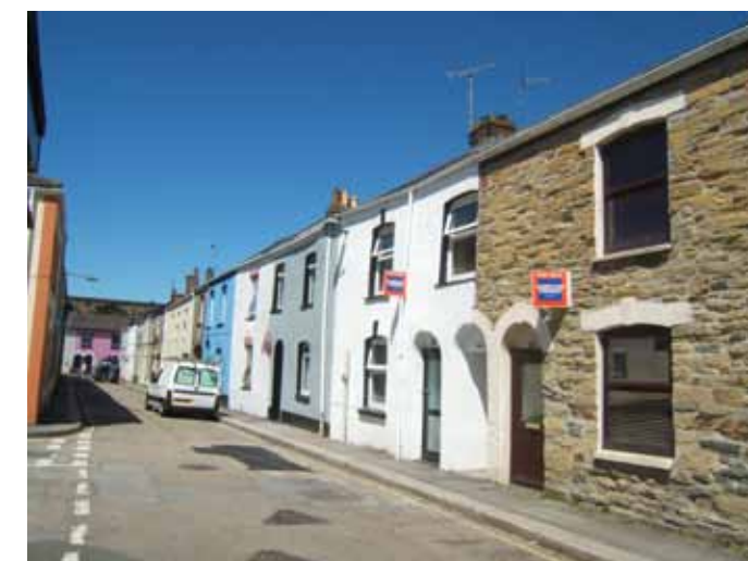
St Dominic Street - The replacement of original windows with uPVC and an inconsistent approach to painting can severely diminish the quality of the street
