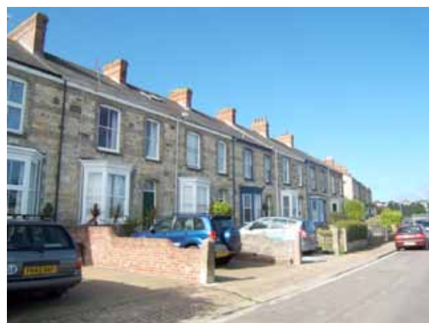
The conversion of front garden areas for parking can undermine the special character of the street- Coronation Terrace
