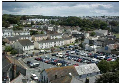
Old Bridge Street car park, dramatic loss of enclosure
