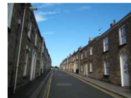
Daniell Street is enclosed on both sides of the street and cuts across the contour running perpendicular to Falmouth Road.
