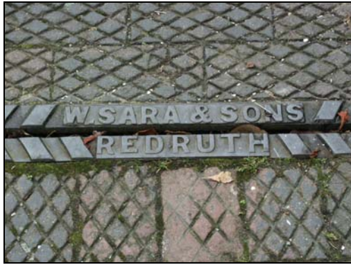
Runnels set in ceramic pavior pavements record the names of local foundry manufacturers
