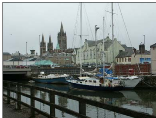
South side of Town Quay
