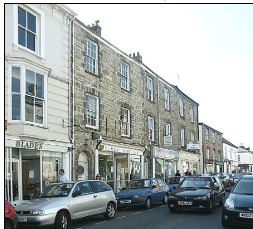
Three-storey former town houses, River Street
