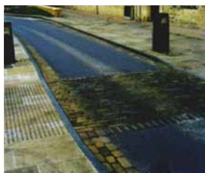
A simple gateway junction that avoids reliance on street markings and signs. Cirencester. (from Streets for All – South West English Heritage 2005)
