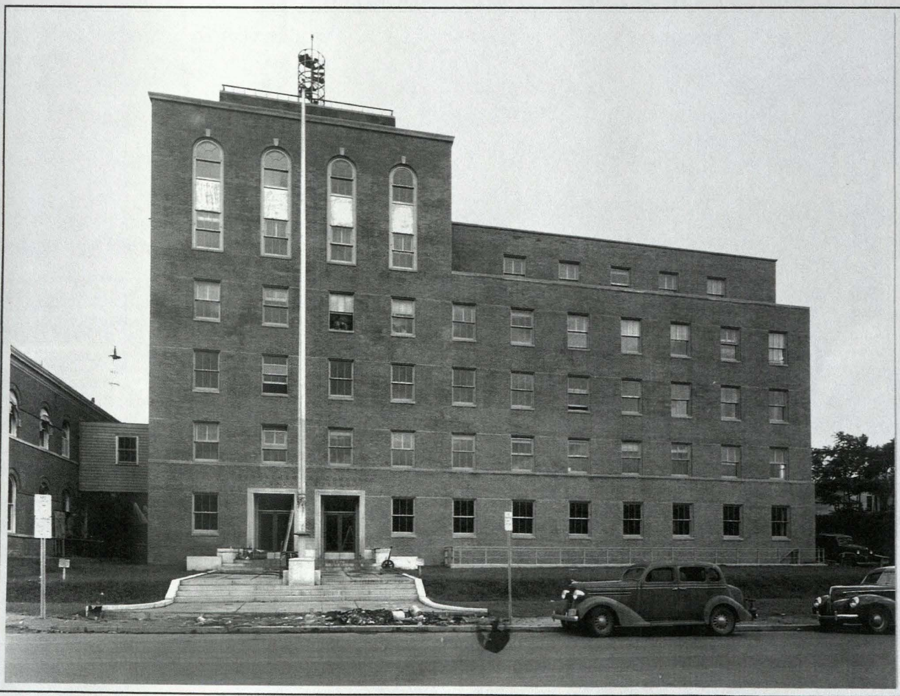
Figure 2. The new 2400 M Street Building.
