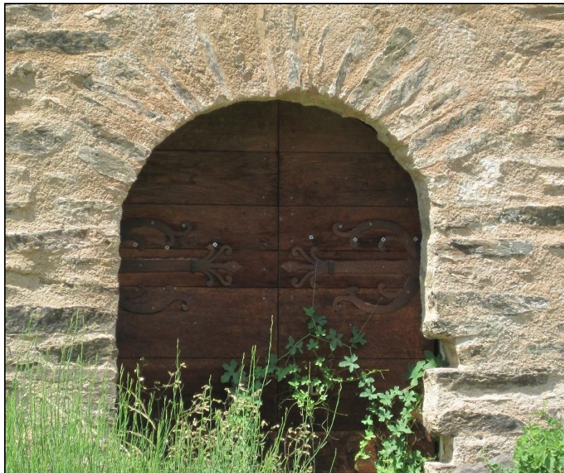
Figure 230: Saint-André de Llar. South doorway.
