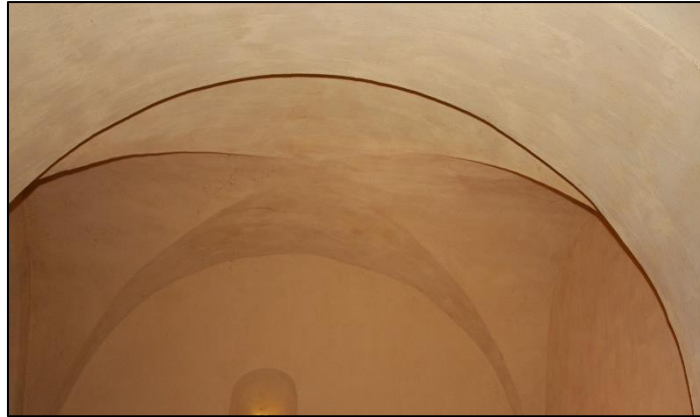
Figure 171: Sainte-Eulalie de Fuilla d'Aval. Interior, south aisle groin vaulting, west bay (detail).
