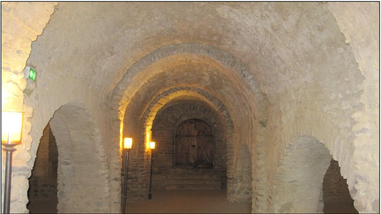
Figure 64: Saint-Michel de Cuxa. Western extension, transverse passage (looking north).
