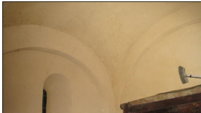
Figure 170: Sainte-Eulalie de Fuilla d'Aval. Interior, south aisle groin vaulting, west bay (detail).
