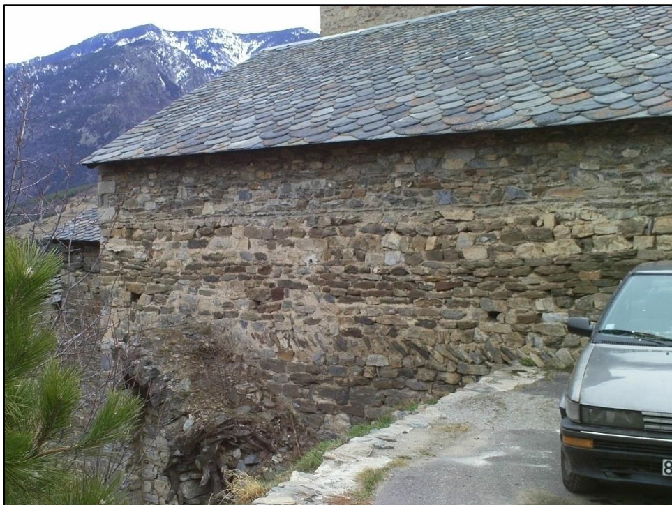
Figure 223: Saint-Martin de Canaveilles. Nave, north exterior wall (detail).
