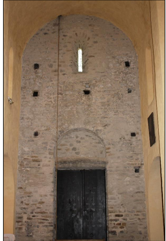
Figure 168: Sainte-Eulalie de Fuilla d'Aval. Nave interior, from east.
