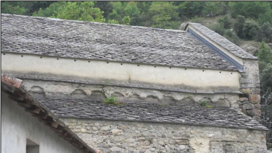
Figure 214: Saint-Jacques de Nyer. South elevation (detail).
