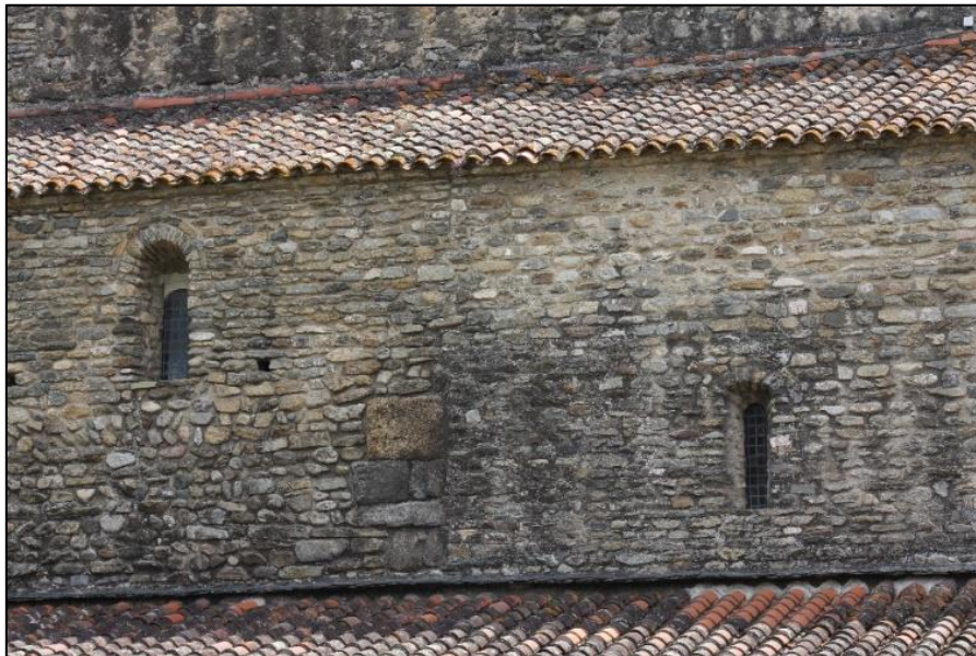
Figure 60: Saint-Michel de Cuxa. North aisle detail.
