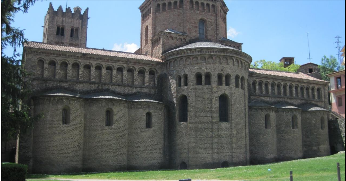
Figure 111: Santa Maria de Ripoll. Eastern elevation.
