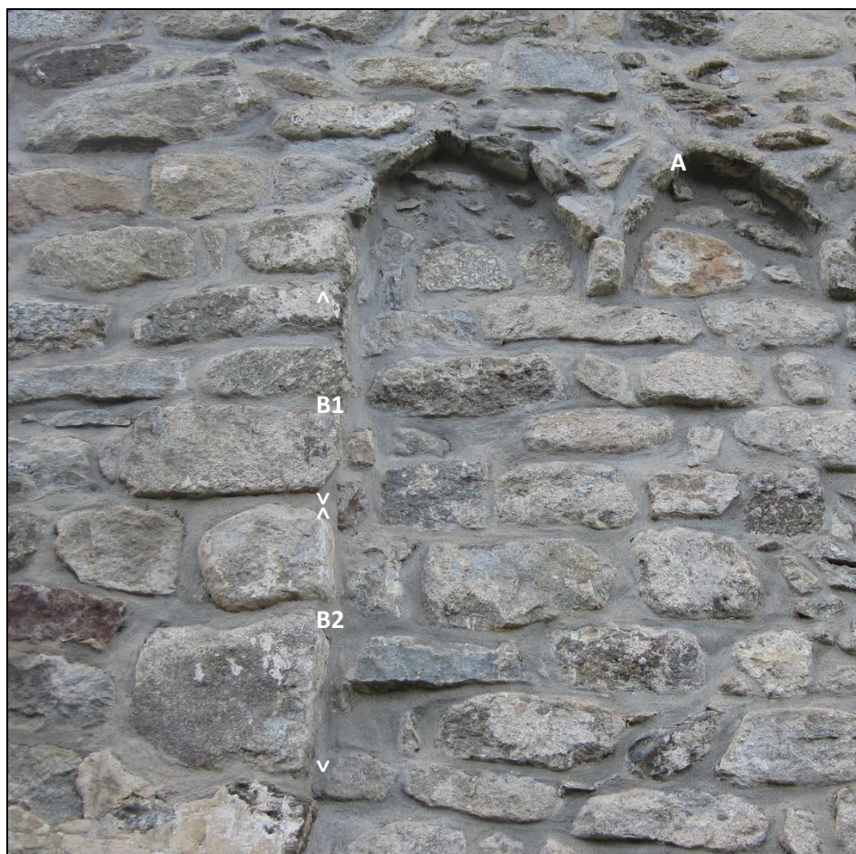
Figure 264: Saint-Paul de Py. South wall masonry (detail).
