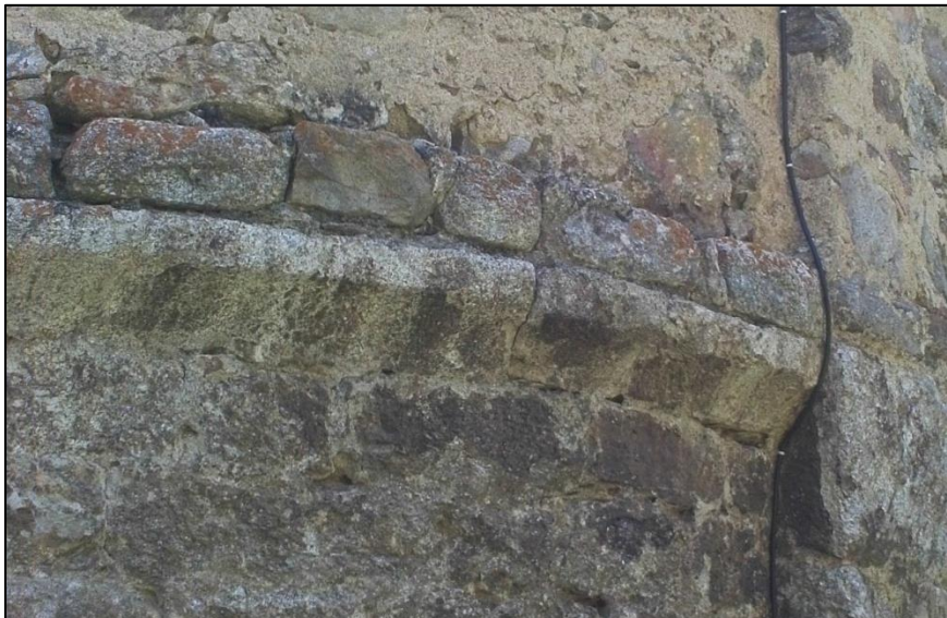
Figure 179: Saint-Vincent de Mantet, apse, original eaves detail.
