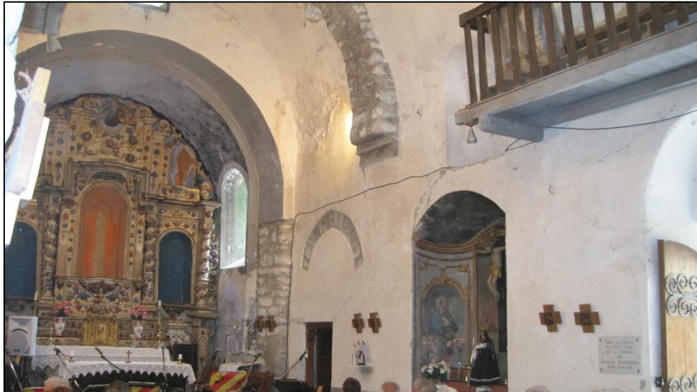
Figure 216: Saint-Jacques de Nyer. Nave interior, from west.
