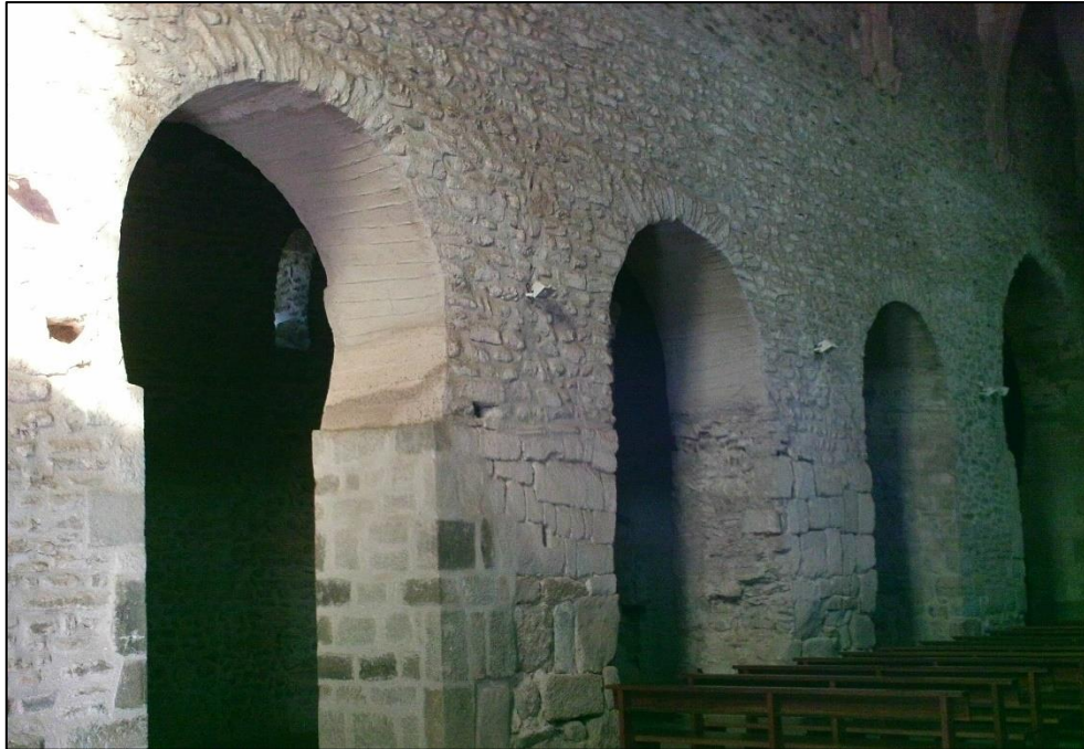
Figure 46: Saint-Michel de Cuxa. Nave, north arcade (from west).
