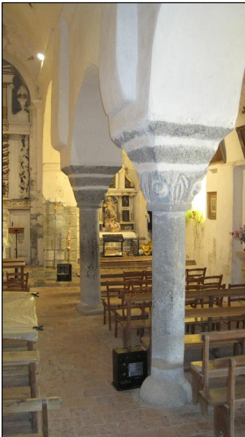
Figure 198: Saint-Vincent d'Eus. Collateral, from west.
