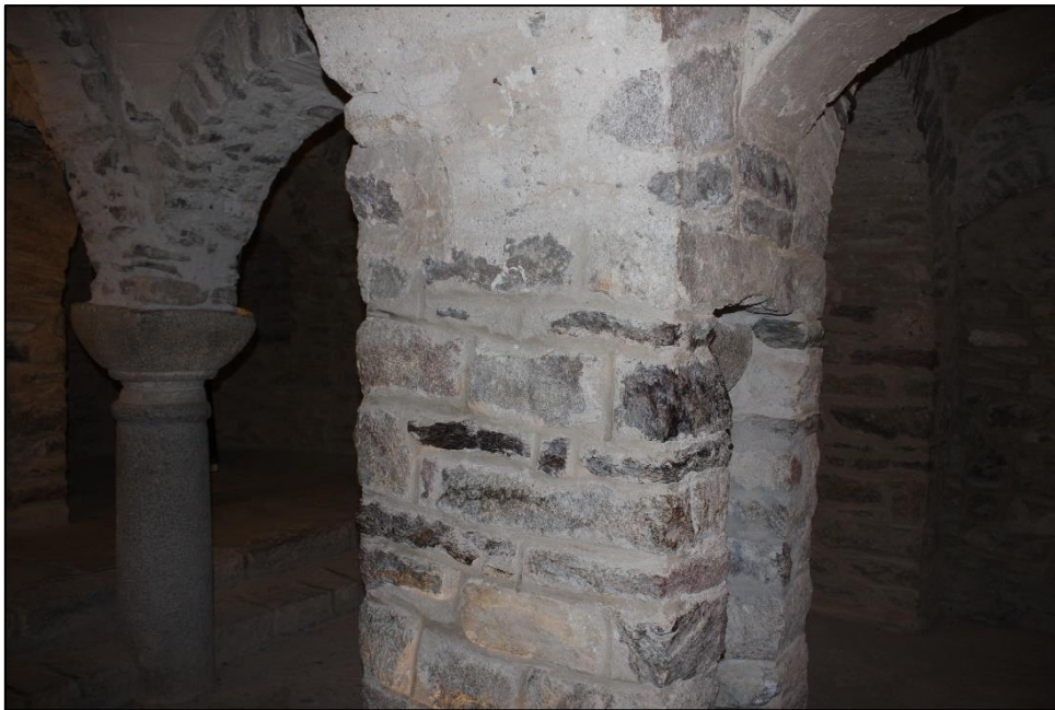
Figure 139: Saint-Martin du Canigou. 'Crypt', eastern section, column & embedded capital.
