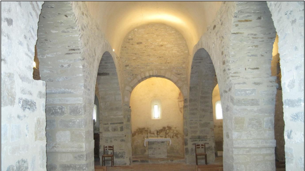
Figure 98: Sainte-Marie de la Cluse Haute. Nave arcades and principal apse.
