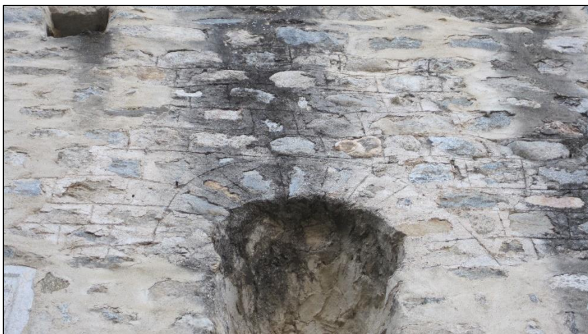
Figure 155: Sainte-Marie de Corneilla-de-Conflent. North elevation, detail.
