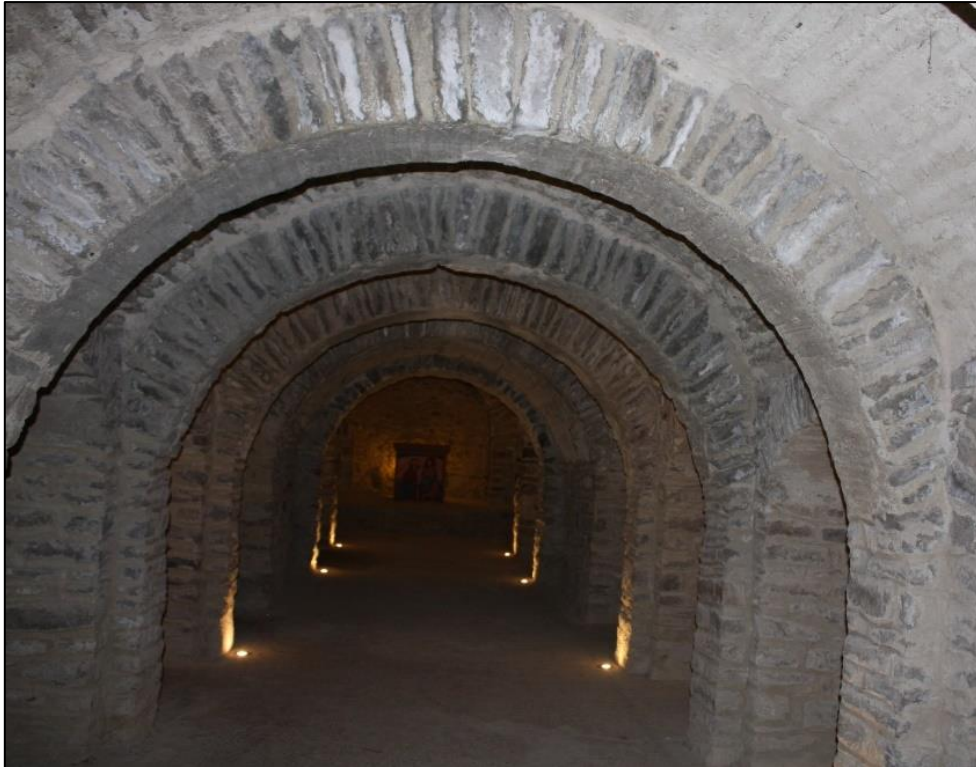
Figure 143: Saint-Martin du Canigou. 'Under-church', central vessel looking east.
