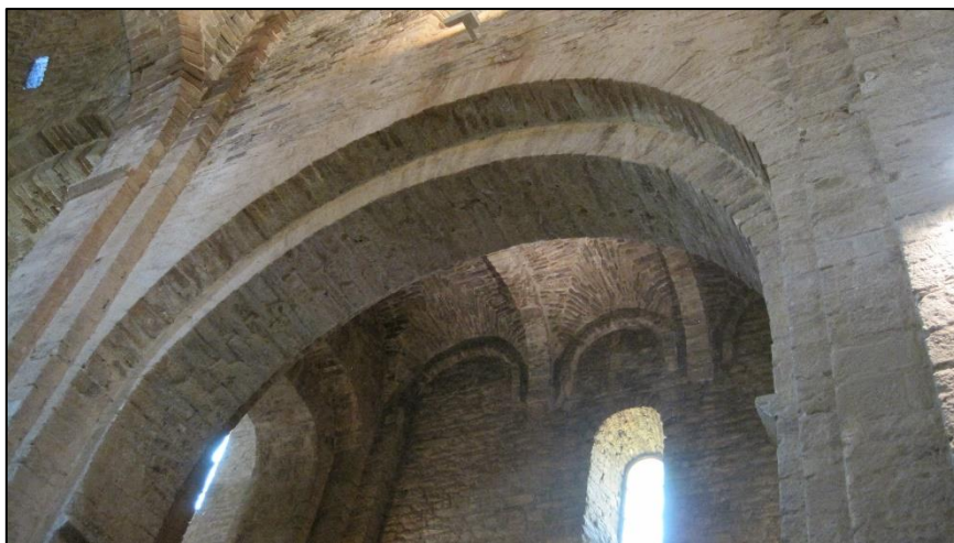
Figure 125: Sant Vicenç de Cardona. Nave arcade and aisle vaulting.
