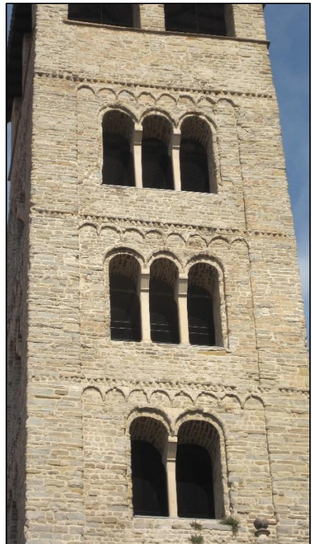
Figure 119: Sant Pere de Vic. Tower detail.
