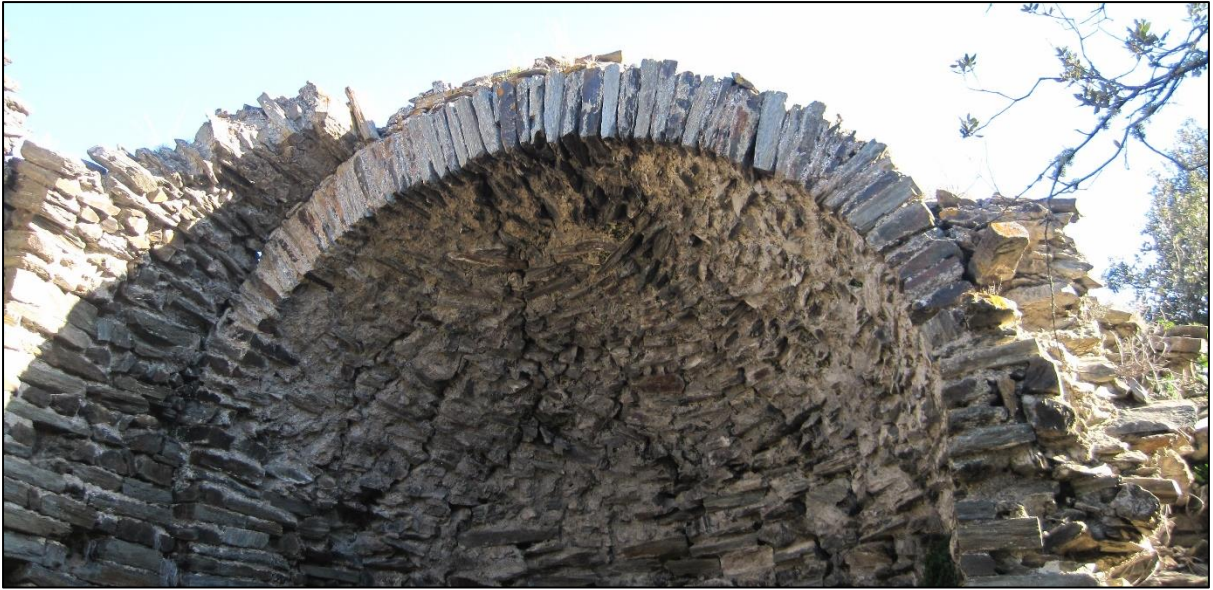
Figure 250: Saint-Étienne de Sofrunys. Apse vault.
