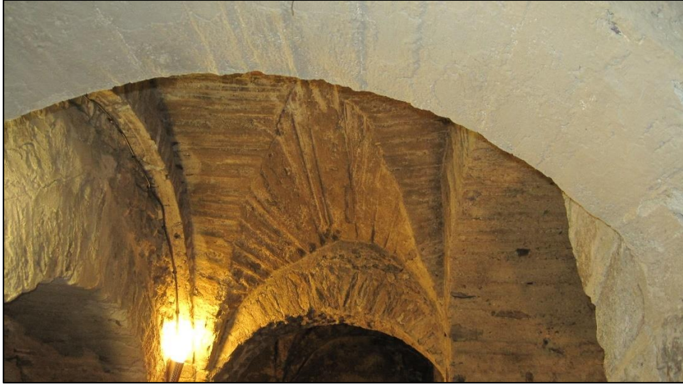
Figure 137: Saint-Martin du Canigou. 'Crypt', groin vault detail.
