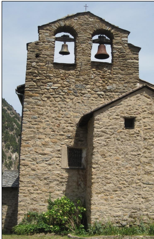
Figure 209: Saint-Génis de Thuès-Entre-Valls. Western elevation.
