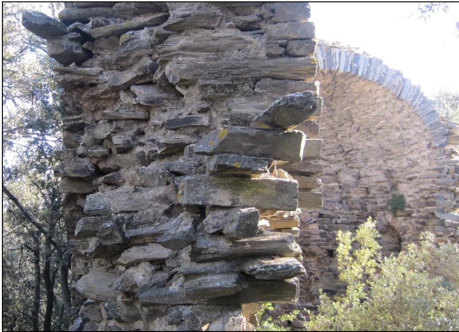
Figure 255: Saint-Étienne de Sofrunys. Masonry (detail).
