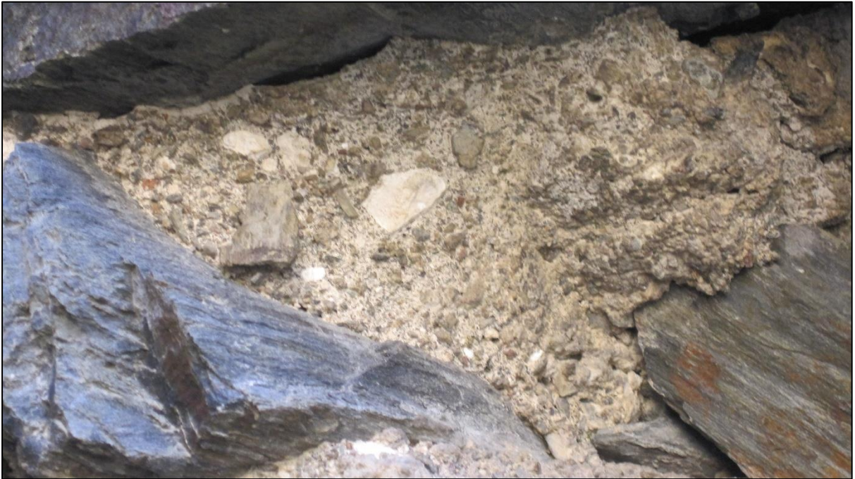
Figure 31: Coarse mortar with rock fragments and unreduced lime nodules, Saint-Étienne de Sofrunys (11 th century)
