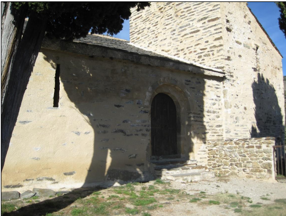
Figure 242: Saint-Julien-et-Saint-Basilisse. South elevation.
