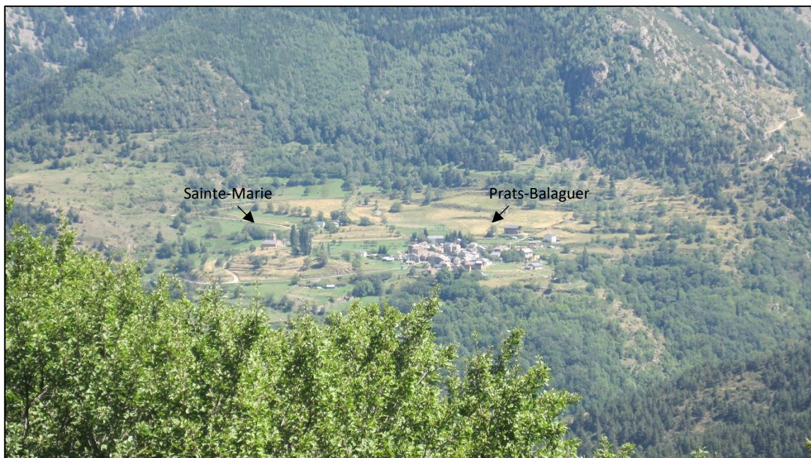
Figure 42: Prats-Balaguer, from north. An example of a parish church lying outside the confines of the village.
