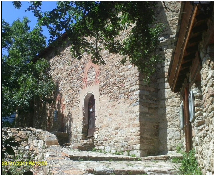
Figure 178: Saint-Vincent de Mantet, south elevation.
