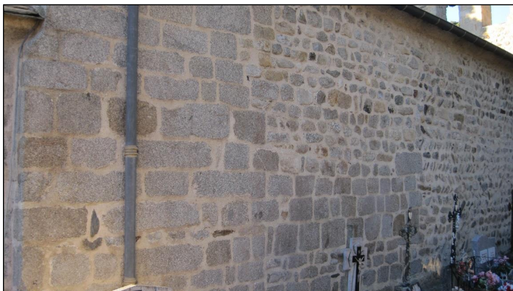
Figure 196: Saint-Vincent d'Eus, north wall fabric (from north-east).
