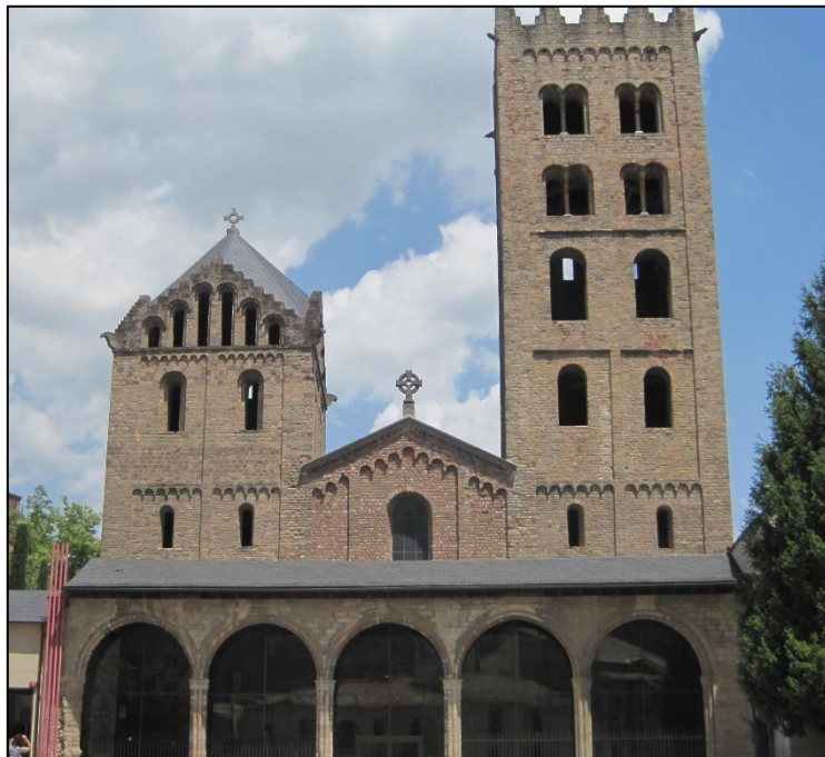
Figure 112: Santa Maria de Ripoll. Western elevation.
