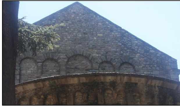
Figure 219: Saint-André de Sorède ( Albères ). Nave wall, east elevation.
