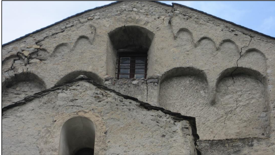
Figure 215: Saint-Jacques de Nyer. Nave, western elevation (detail).
