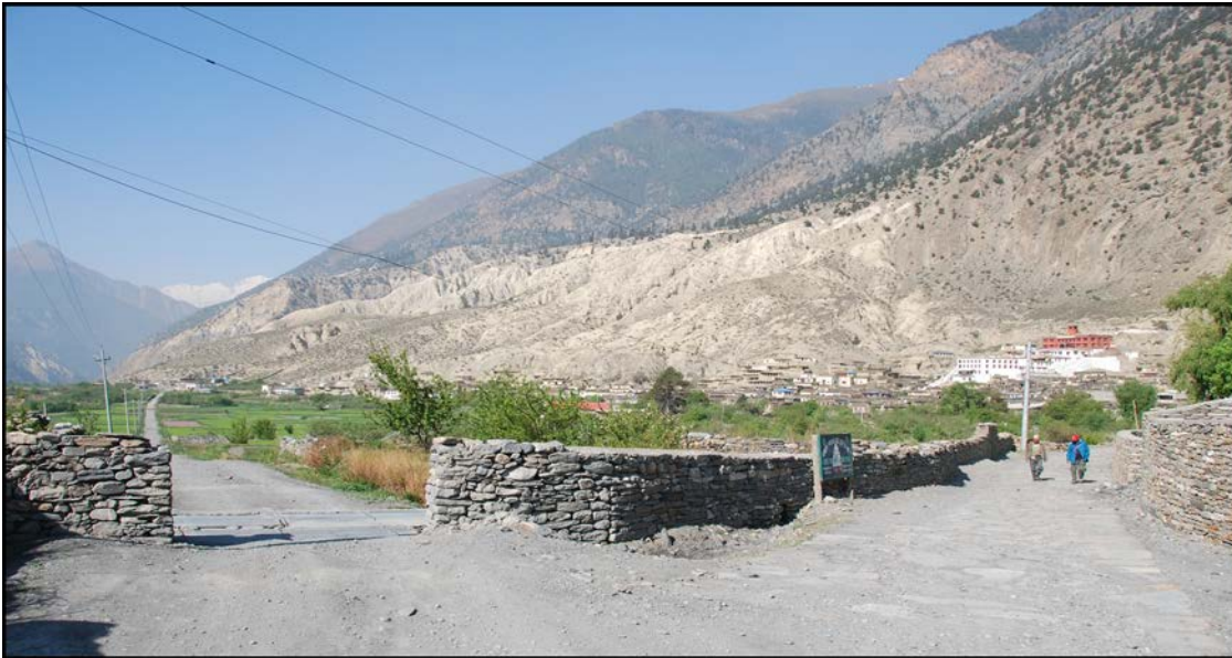
Figure 4.44 The conjunction of the Kali Ghandaki Road (left) and the ACT (right) on the north side of Marpha (R.E. Beazley 2009)
