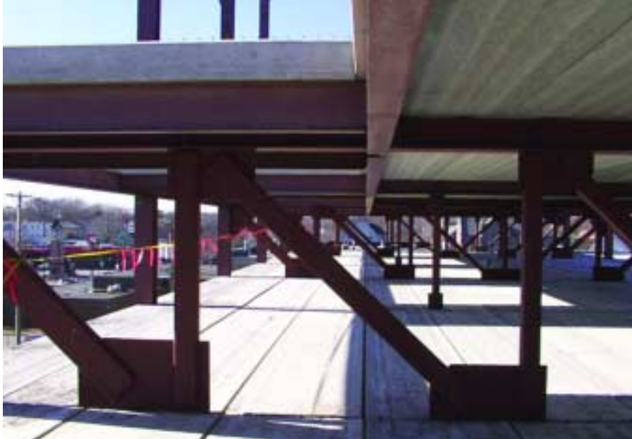
The Legacy Towers' mezzanine loft approach is probably the first of its kind for staggered-truss construction. At each mezzanine floor, the pre-cast concrete floor planks are removed within the interior of the floor plan. This allows each apartment to have a two-level occupancy, where tenants access the mezzanine from their main floor via staircases.
