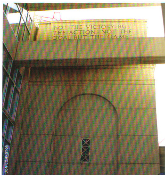
The most memorable quote at Memorial Stadium is hidden behind newer construction on the west side. To see it, you need to look up.
