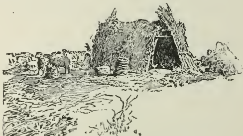
ARAB WORKMAN'S HUT.
